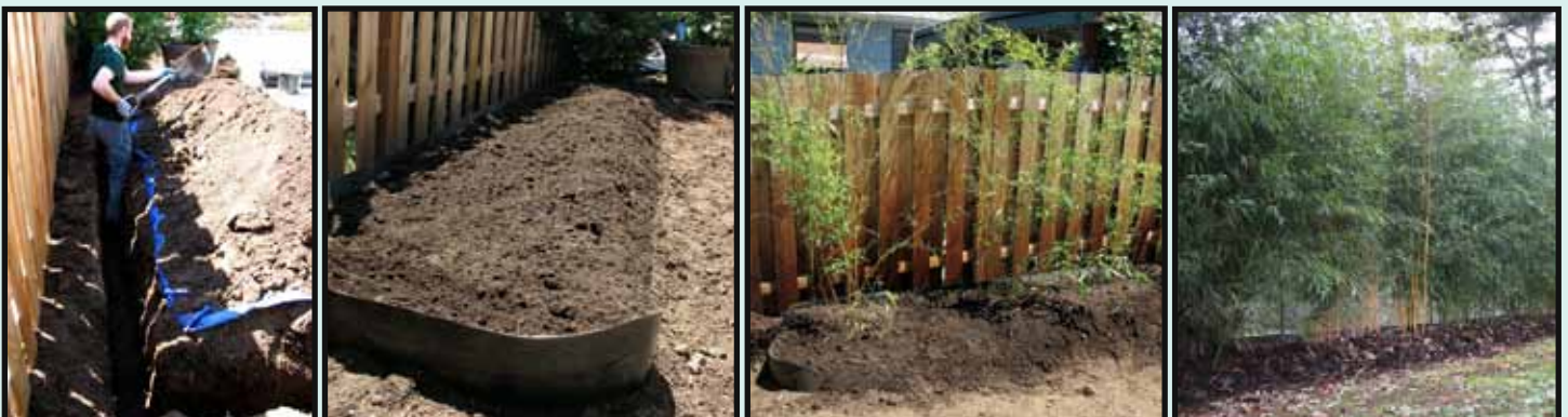
Left to right: 1. A 28" deep trench being dug for barrier. 2. Installed barrier with a berm. 3. Young bamboo planted in berm. 4. Bamboo in same planting area a few years later.
